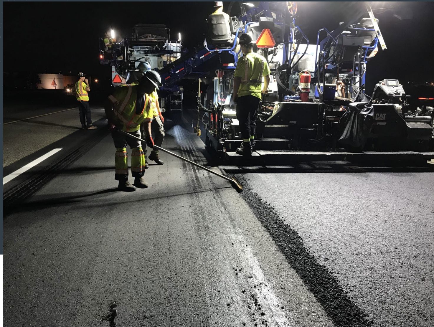
Paving 2nd Pass
