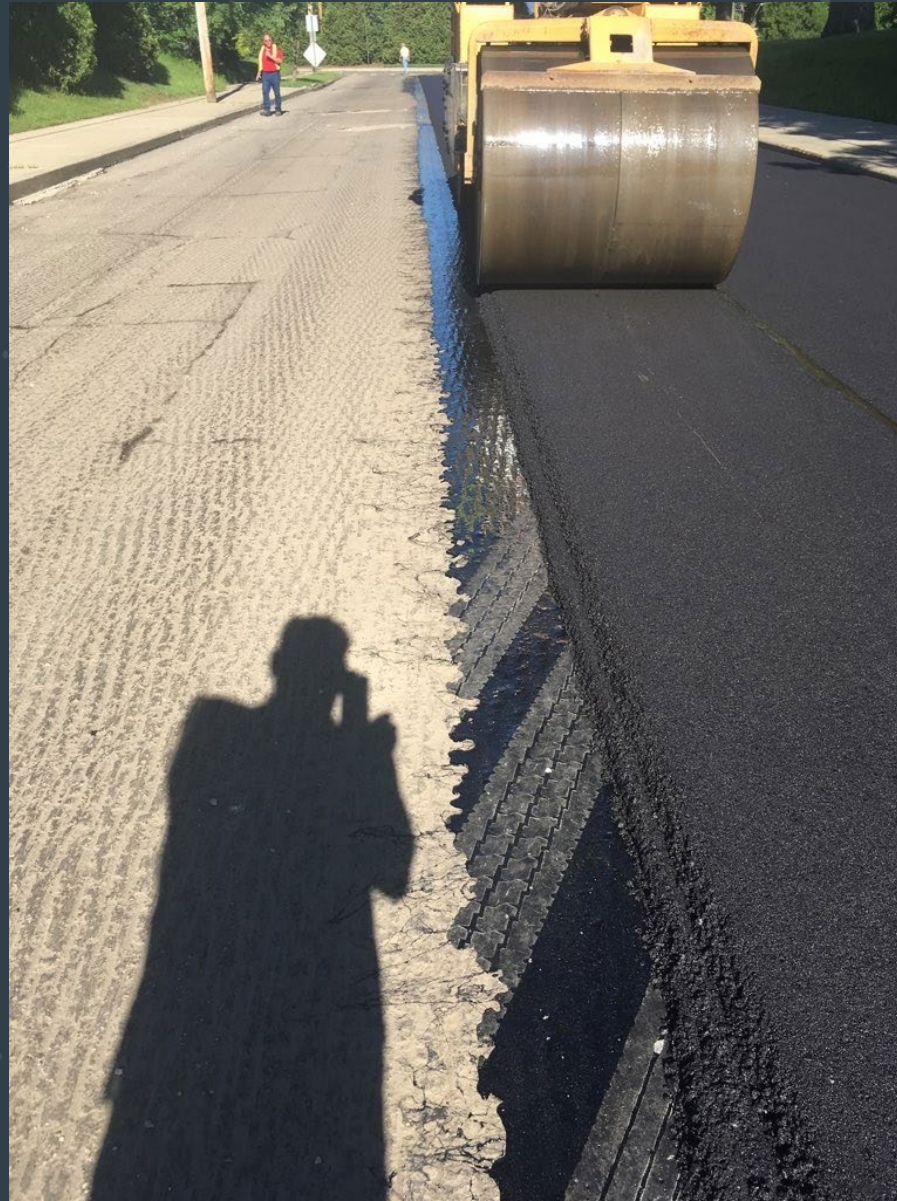
1st Roller Pass Overhang Joint
