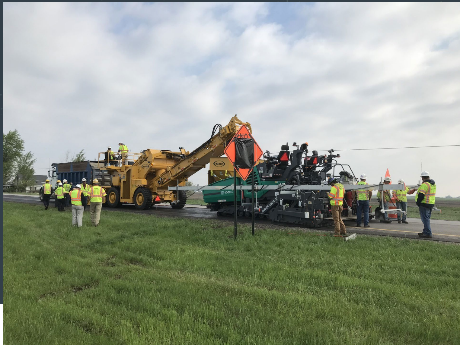
Paving 2nd Pass
